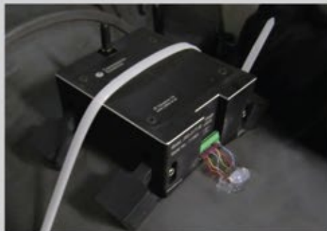
Completed mounting - ready for startup
